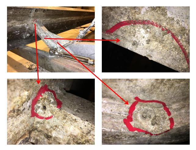
Figure 2: Skimmer Arm Corrosion
