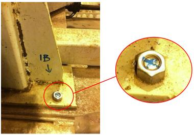
Figure 4: Bolt with Inadequate Length
