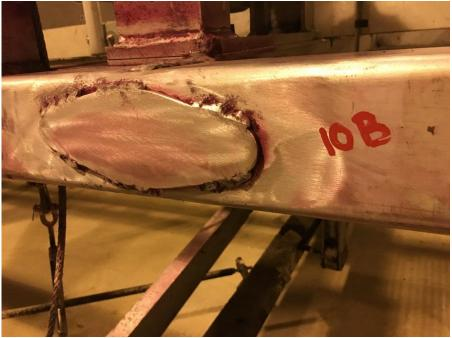
Photo of fish plate at location 10B. Poor weld quality
