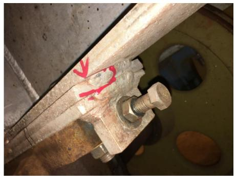
Cracked bearing mount plate weld at location 1B
